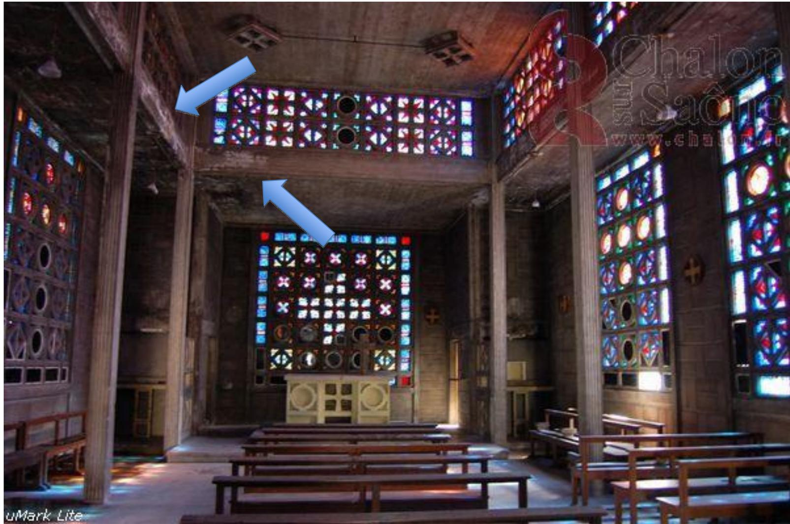
Chappelle de la Colombière – Water percolating inside the concrete envelope, pinpointed by efflorescence. Potential risk of damaged structures for the thenardite-mirabilite cycles. Hypothesis to be verified.
